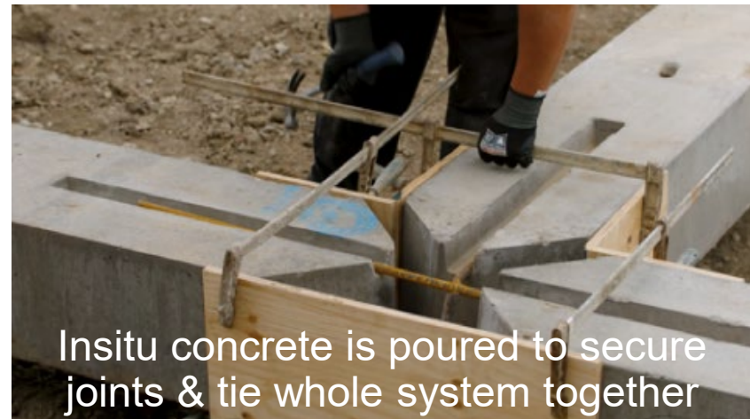
Beams are laid onto the caps
