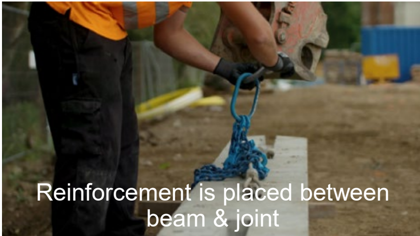
Precast Caps are placed onto pile using bedding mix
