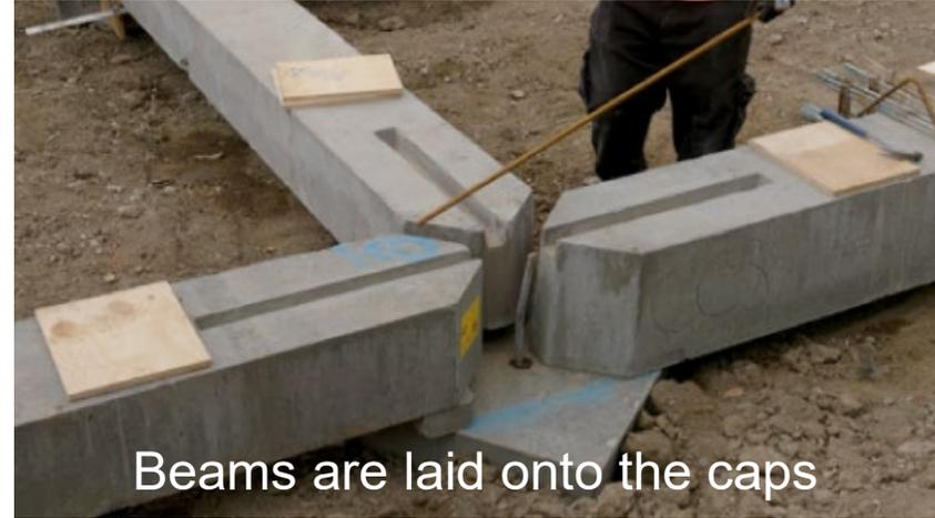
Beams are laid onto the caps
