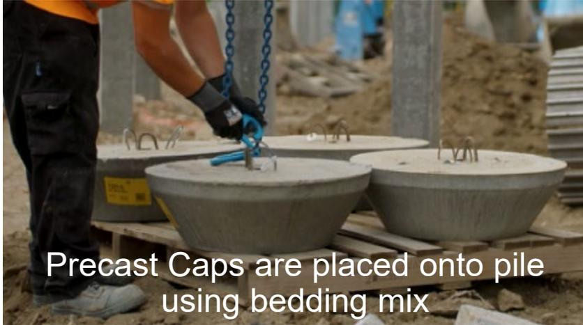
Precast Caps are placed onto pile using bedding mix
