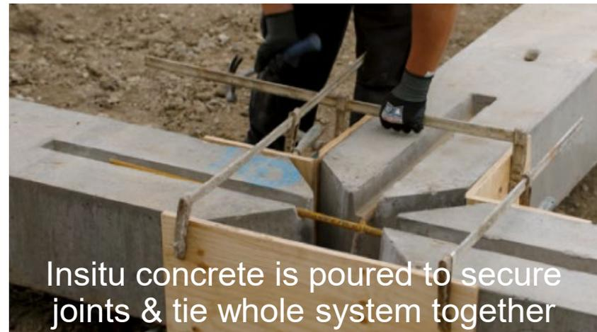
Insitu concrete is poured to secure joints & tie whole system together
