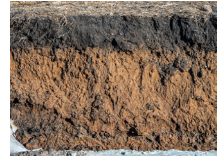
Irregular mass backfill
