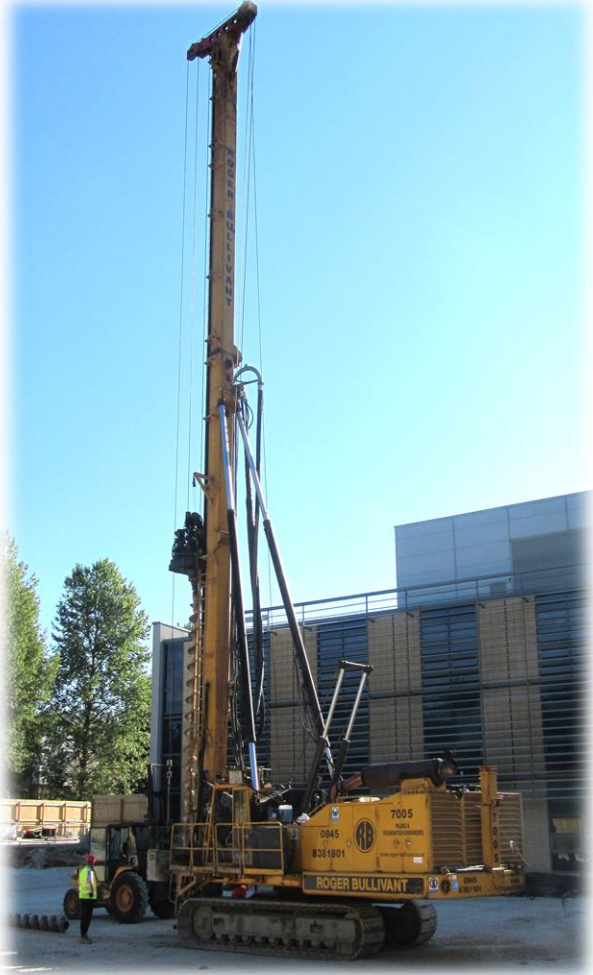
Continuous Flight Auger (CFA)
