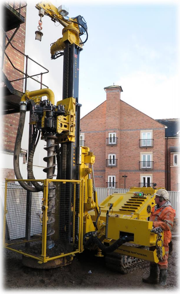
Sectional Flight Auger (SFA)
