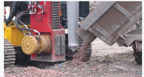
1. The steel vibrating probe is inserted into the soil to the required depth. The vibrations from the probe densify the soil which creates a void.
