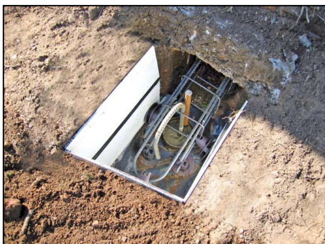
Preparation completed - Ready to pour
