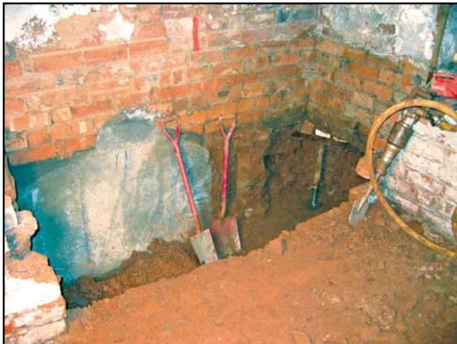
Preparation to a corner section of a basement
