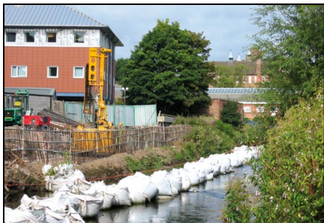
1 Flood Defences - Docks - Harbours
